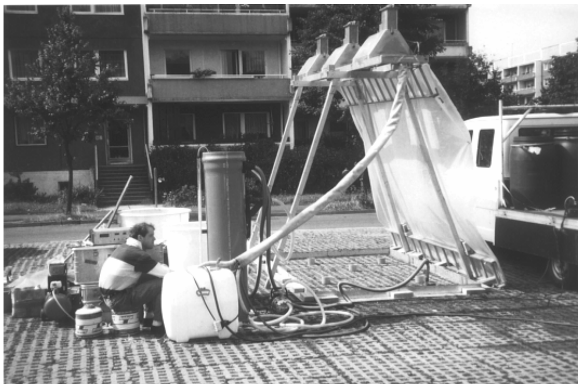
Figure 2. Measuring the permeability of a sealed soil covered by concrete plates with drainage openings using a portable rainfall simulator
